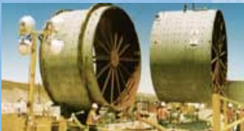
Welding a mill shell on site.
