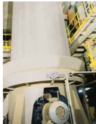
Drive unit of the fines cooler.
