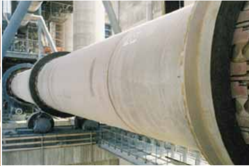
Rotary kiln supported on 3 roller stations.
