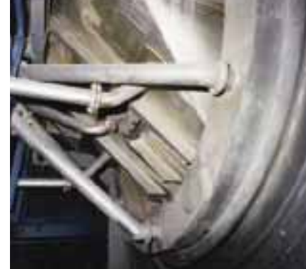
Air-cooled kiln inlet trough.
